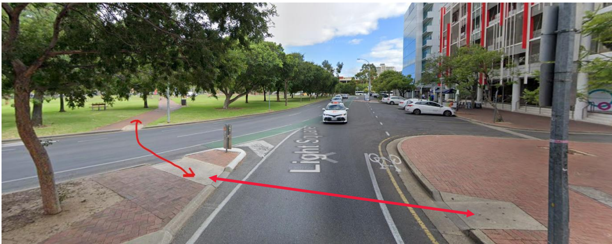
One crash involving a pedestrian, resulting in a minor injury, was reported during the most recent five-year period at the southeastern unsignalised pedestrian crossing. Refer to Section 4.6 for historical crash data analysis.
